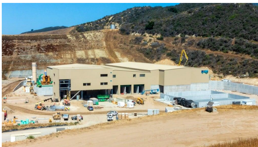
Figure 16: The Tajiguas Landfill in Santa Barbara is adding a MRF and anaerobic digestion for organics, which is expected to extend landfill life by about a decade 27 .
