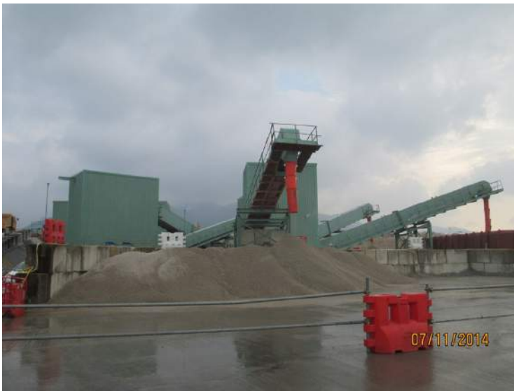
Figure 2 The crushing plant with material segregation
